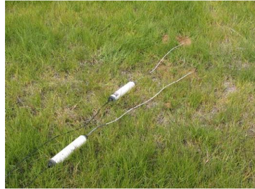
Buried sensors connected to smart interface
