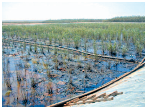
Reed bed treating process water (left) and treated water outflow (right)
