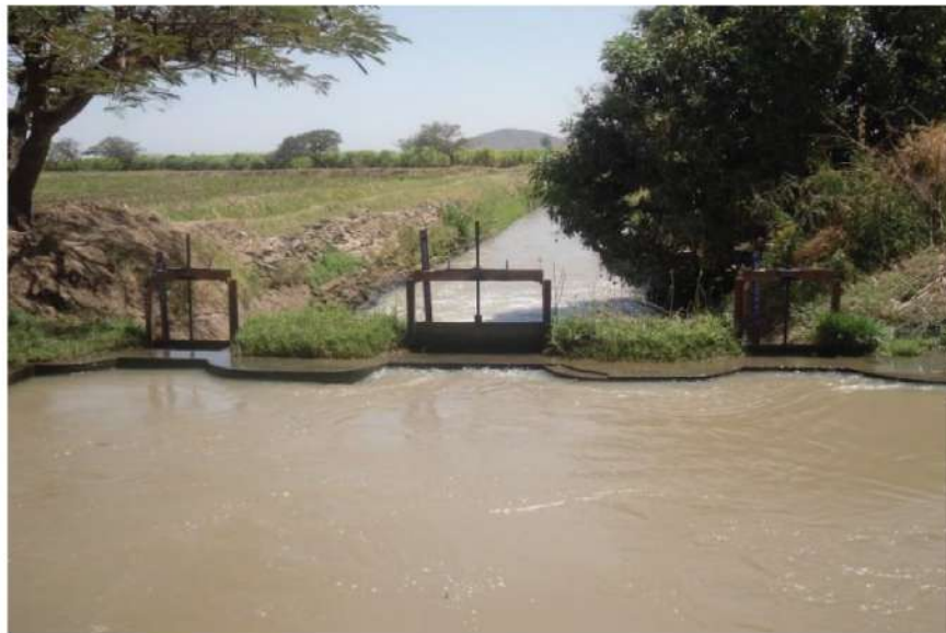
Conveyance and flow control systems of the modern public irrigation scheme
