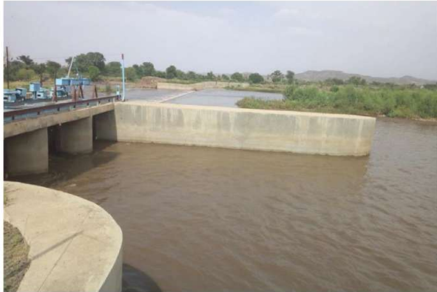
Headwork for a modern large scale community irrigation scheme
